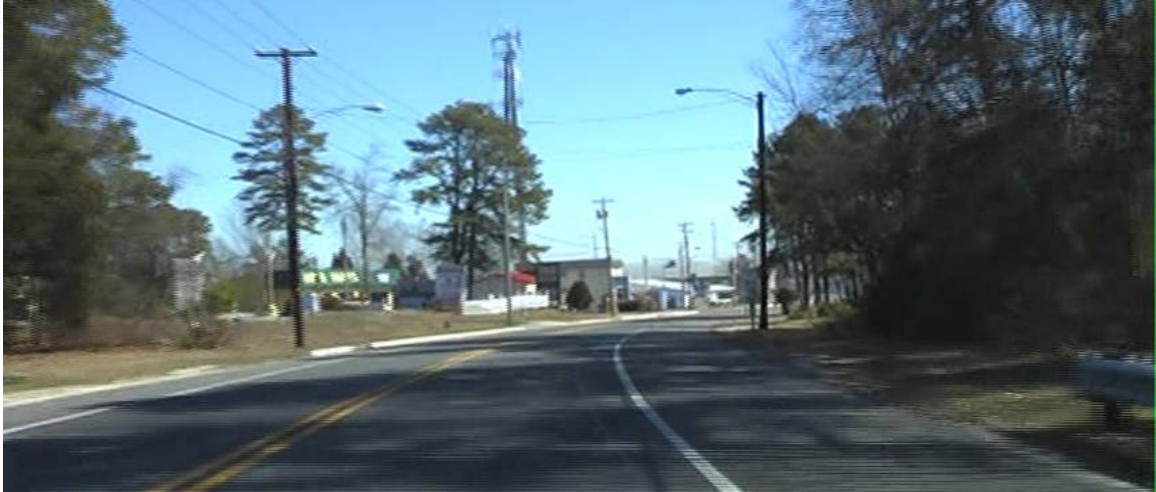
US 9 approaching Giffordtown Lane, Little Egg Harbor Township – Pinelands Regional Growth Area
